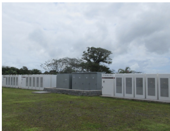
Figure 16: BESS at Fiaga Power Station
