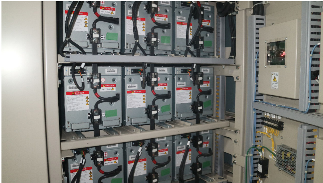
Figure 23: 0.5 MW BESS at Popua Power Station
