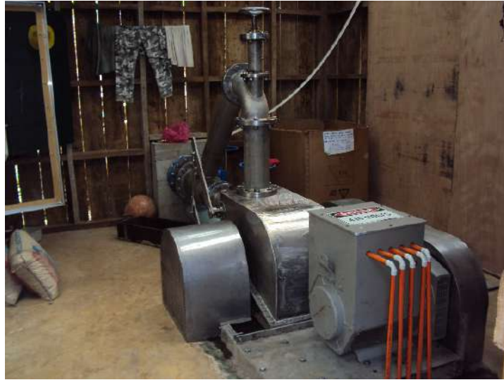
Figure 15 A picture showing a micro hydro range turbine-generator installation Source: Pelena Energy
