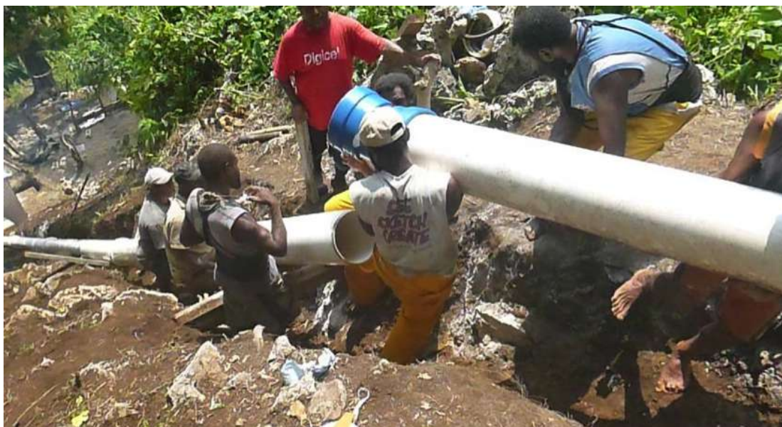
Figure 8 Penstock Installation works in Vanuatu Source: Pacific Regional Data Repository (PRDR)
