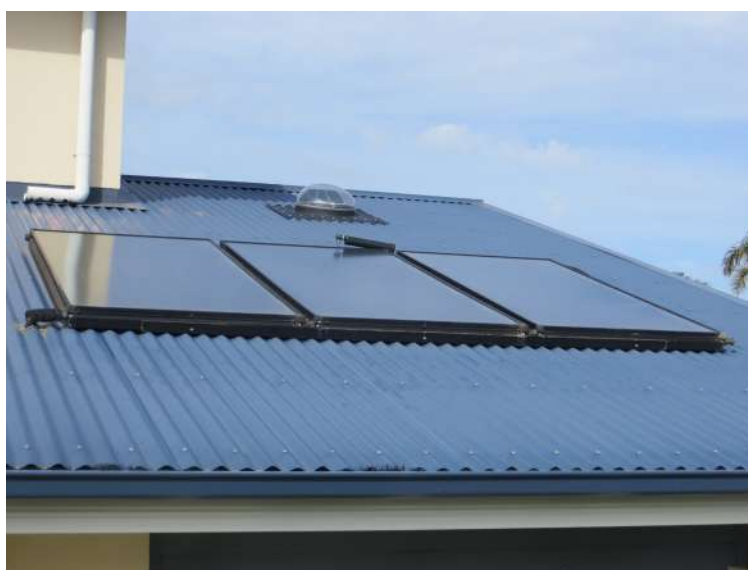
Figure 6: Flat-Plate Collector Photo
