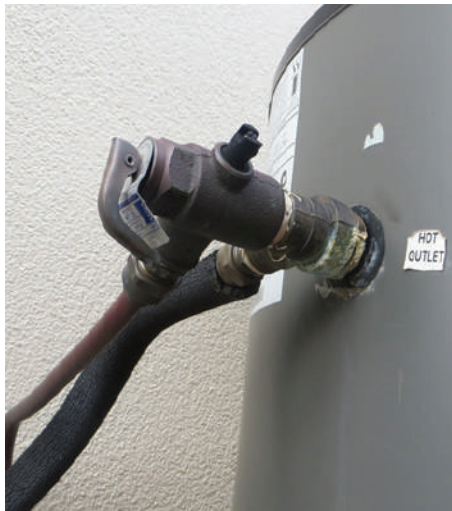
Figure 27: TPR (Left) and Thermostatic Mixing Valve (Right), Showing Ample Accessibility
