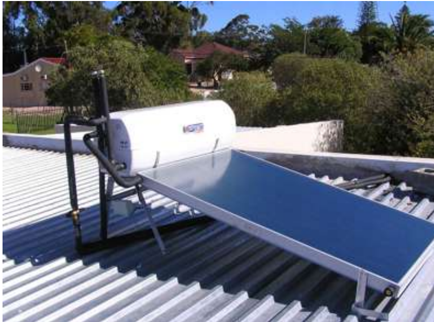
Figure 13: Typical Installation On A Flat Roof
